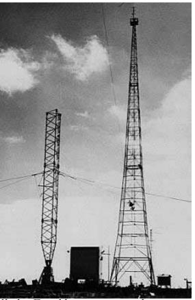
KNBC (KPO)'s present 550 ft. tower was completed in 1949. This type of antenna is called a Franklin antenna, a design used by only a few AM stations in the U.S. The antenna is easily recognized by the porcelain insulator in the middle of the structure.
